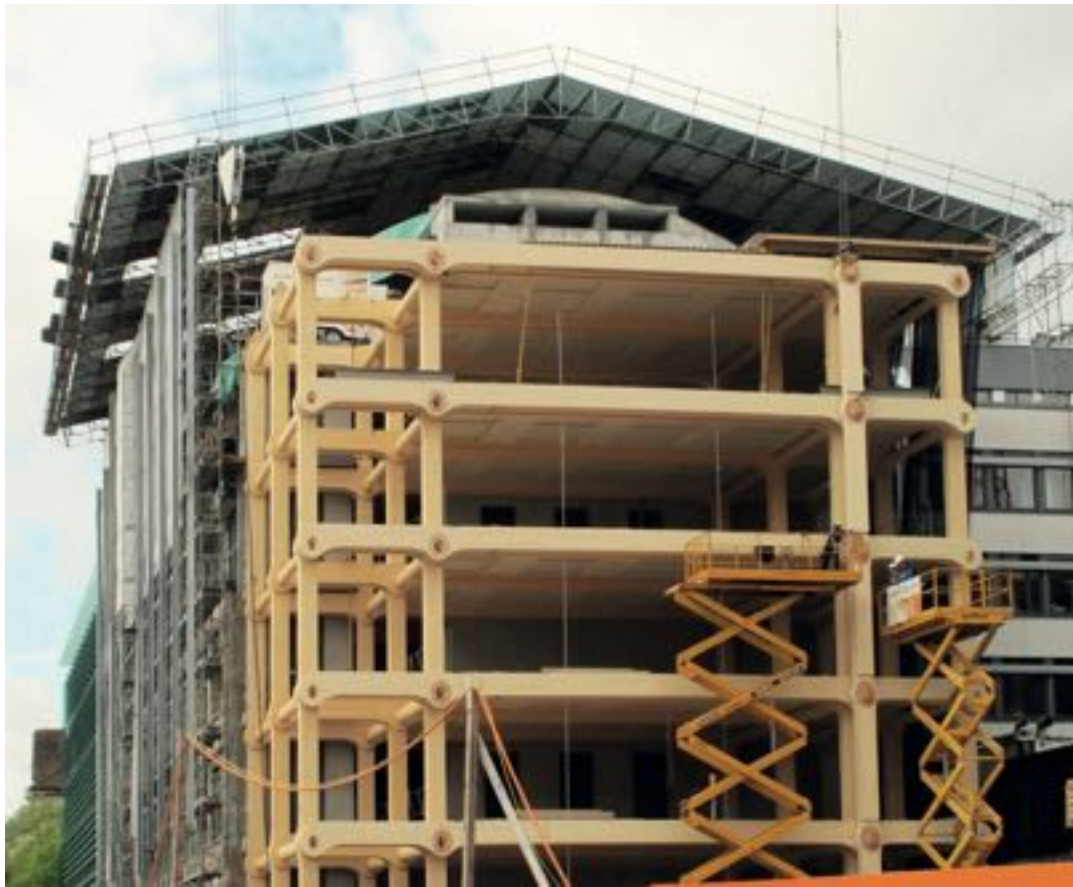
The structure of the Tamedia Office Building, in Zurich, is realized with 2000 m3 of wood.
